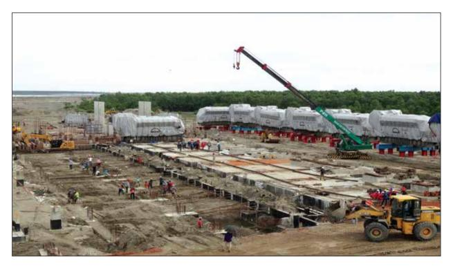
Placement of Engine of Mirsarai 150MW Power Plant on Engine Bed
