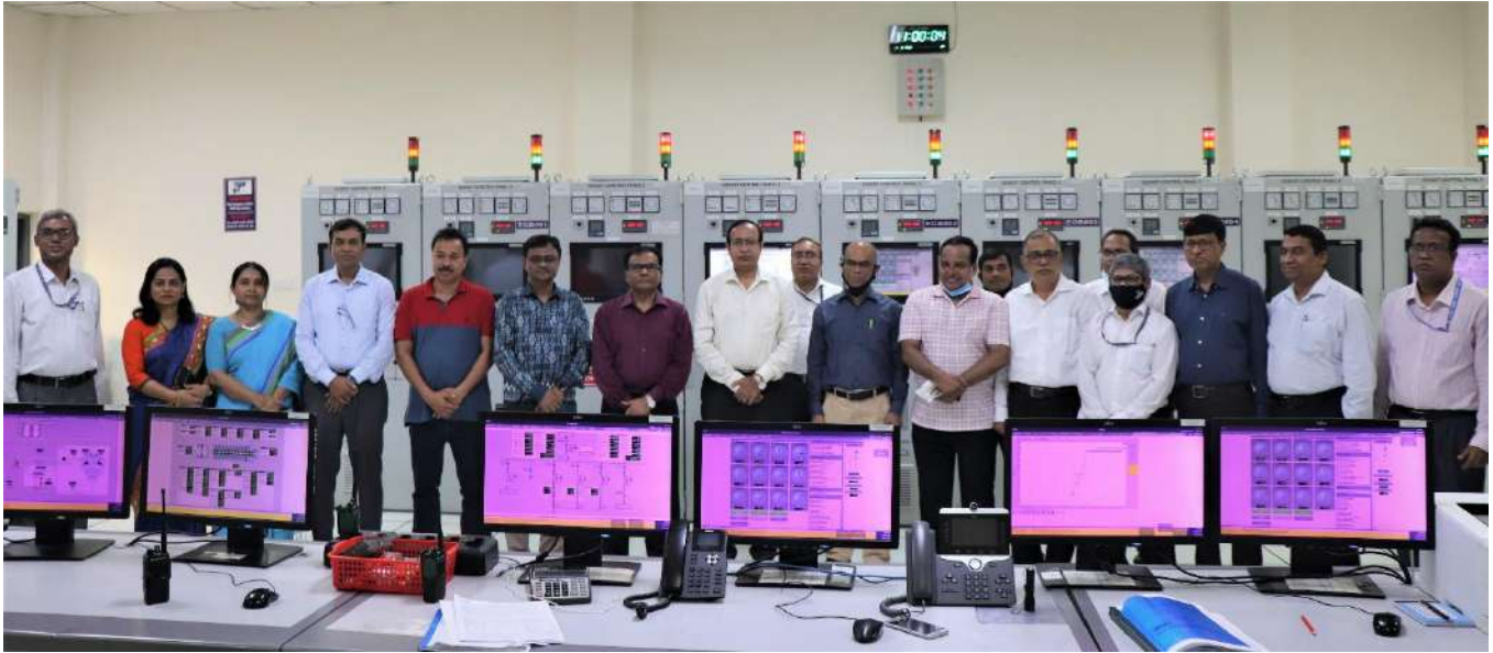
The Hon'ble Secretary, Power Division and the Chairman of BPDB & BRPL with other high officials at Control Room of Kodda 150 MW Power Plant
