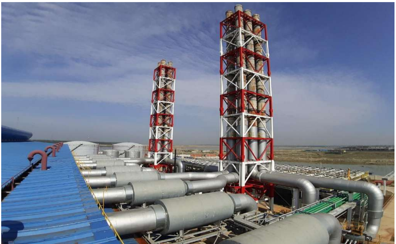
Stack & Chimney of Mirsarai 150MW Power Plant Project
