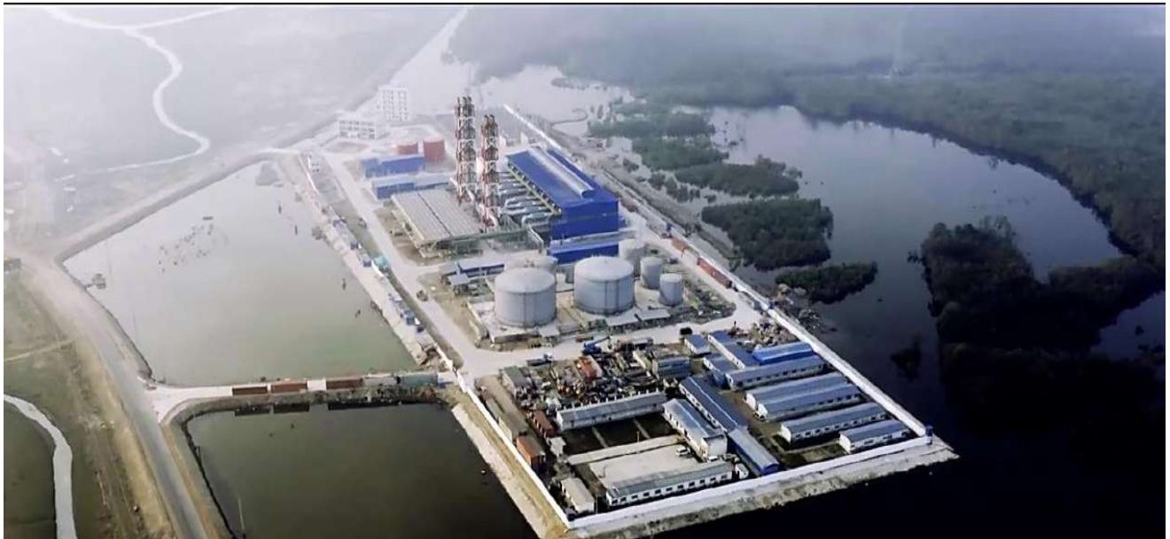
Overview of Mirsari 150 MW Power Plant Project
