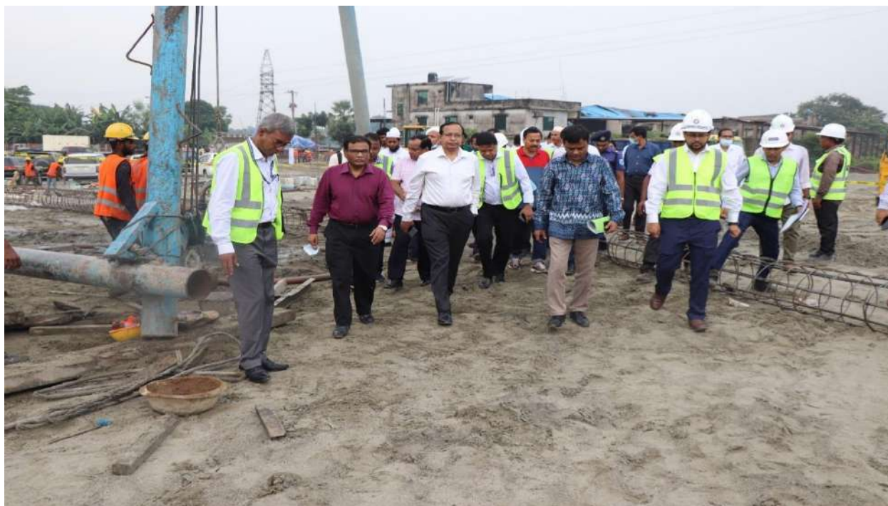
Secretary, Power Division and Chairman, BRPL along with Managing Director visited Sreepur 150MW HFO Based Power Plant Project.
