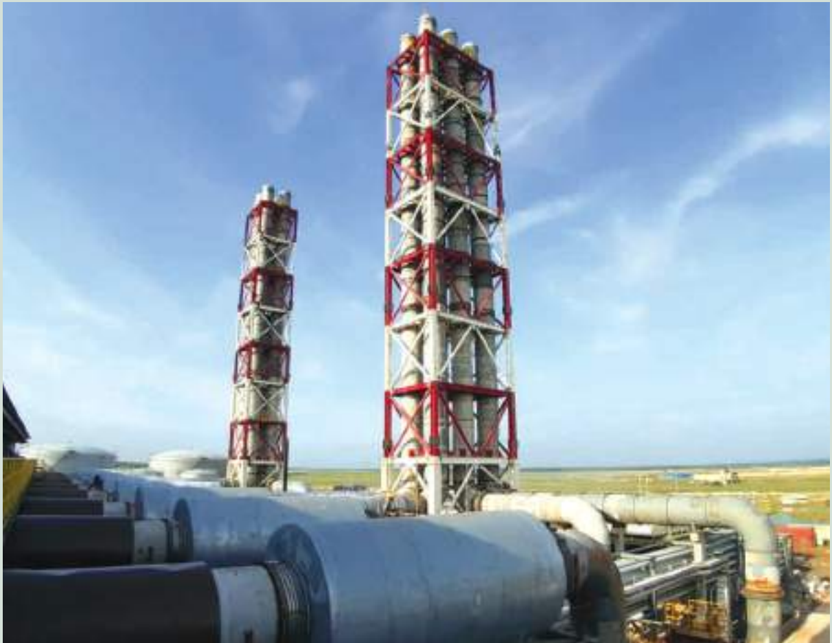
Exhaust ducts on Mirsarai 150 MW Power Plant Project
