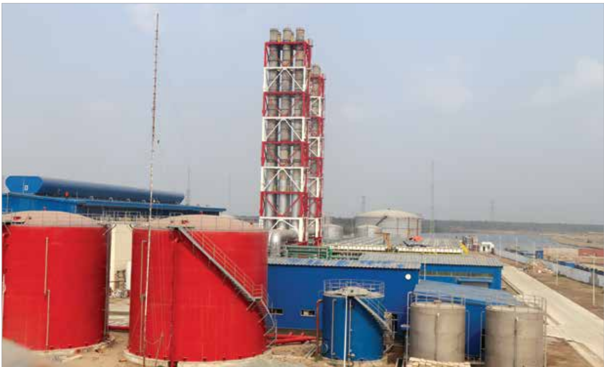
Mirsarai 150MW Dual Fuel Power Plant Project Overview
