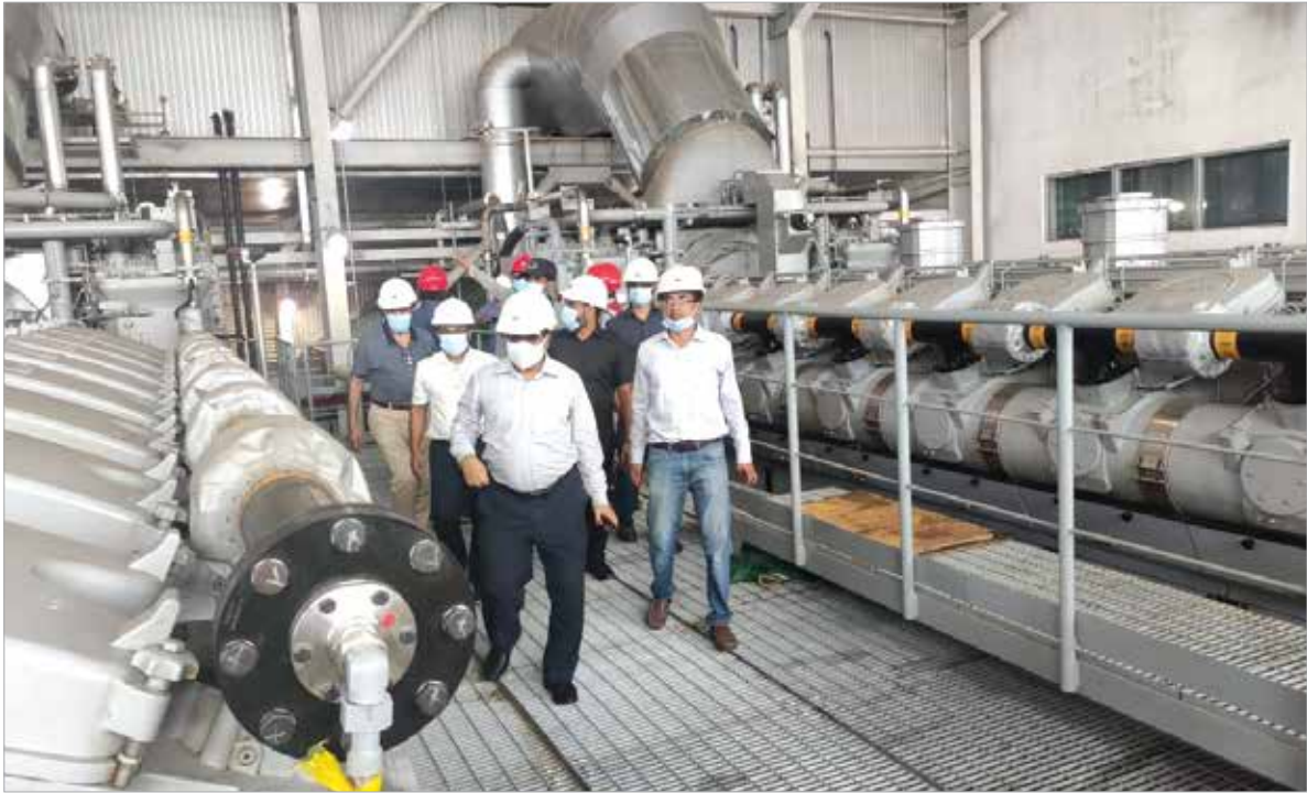
Hon'ble Chariman Visits Mirsarai 150MW Dual Fuel Power Plant Project
