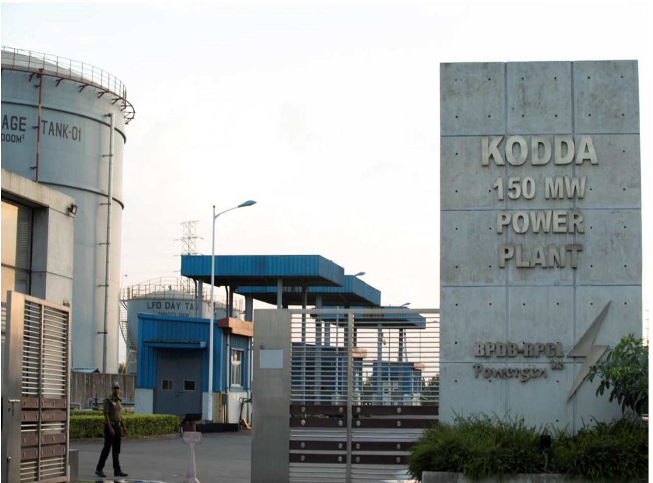
Kodda 150 MW Power Plant, BRPL
