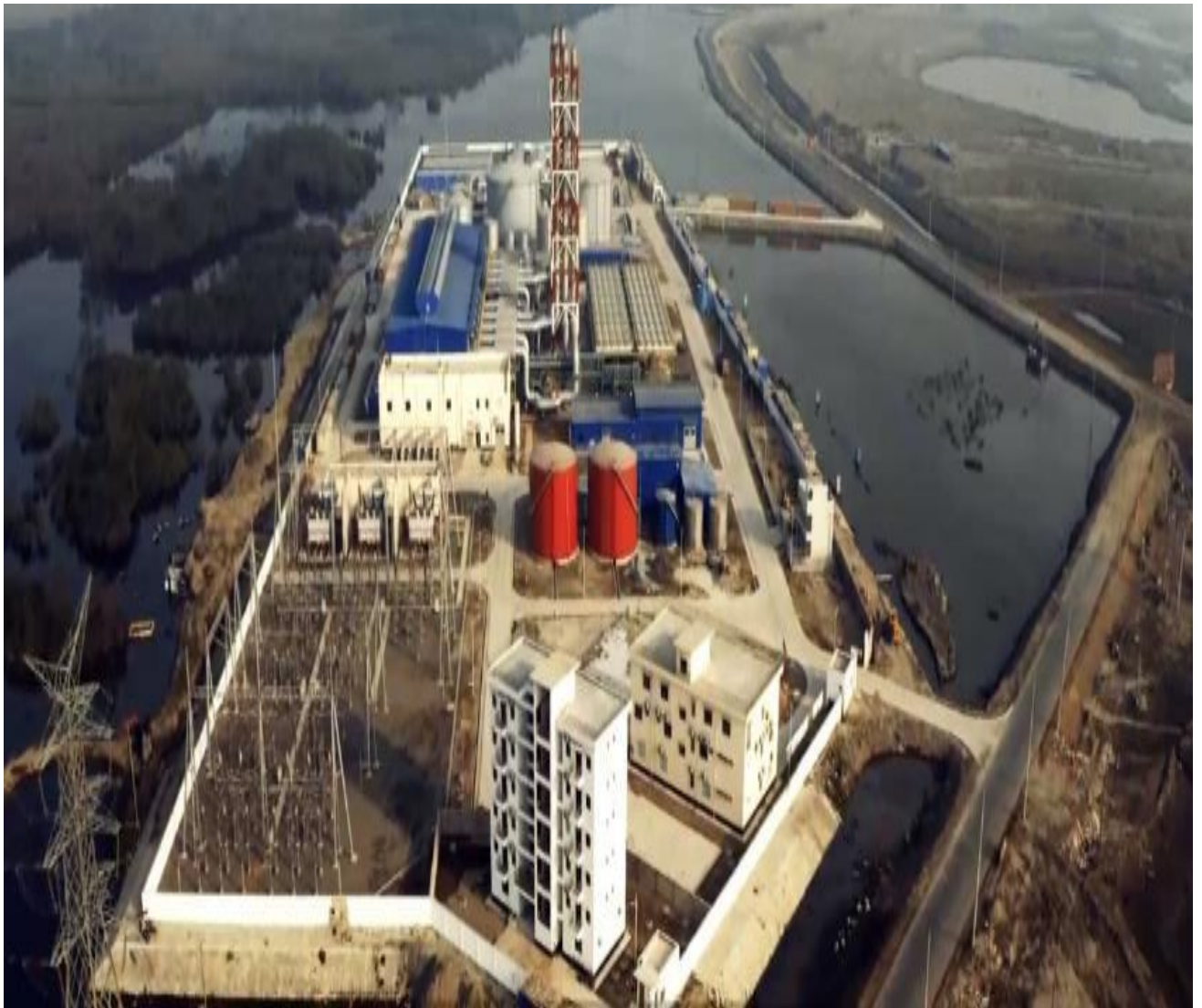
Mirsarai 150 MW Power Plant Project
